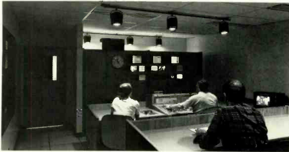
Track lighting in production control keeps light off Sony and Panasonic monitors and focuses it on work areas.
