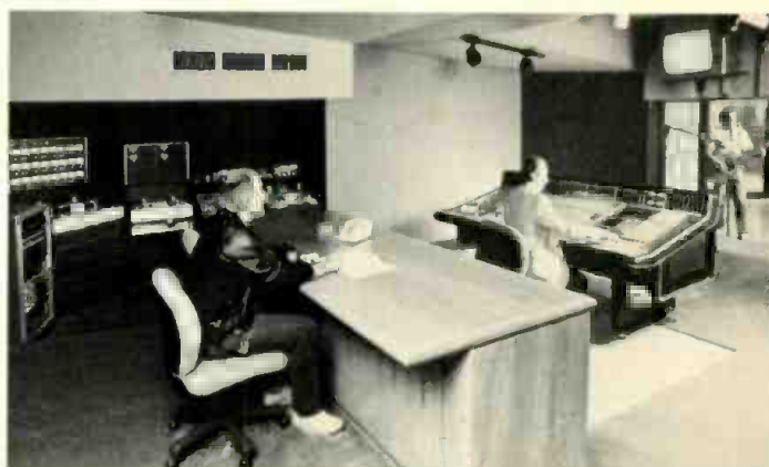
A complete audio recording studio allows full sweetening functions with an SSL 6000E console, Eclipse synchronizer, and Studer multitrack recorders.
