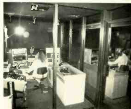
Sliding glass doors allow full visibility of all studios at KWVE-FM.
